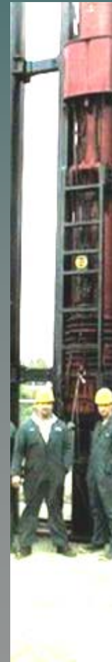
APE D62 produced less noise. Energy was slightly lower.
